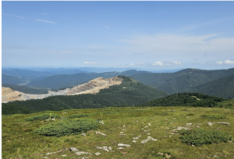
Murgana: site view
