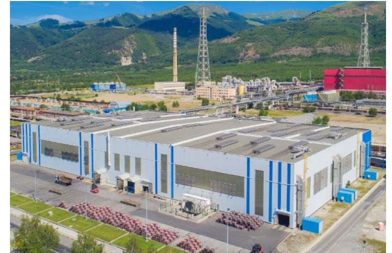
Aurubis: infrastructure view
